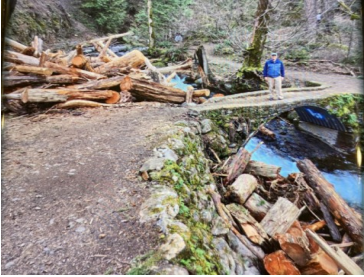
Upper Multnomah Creek Bridge February 2026 Photo by a hiker
